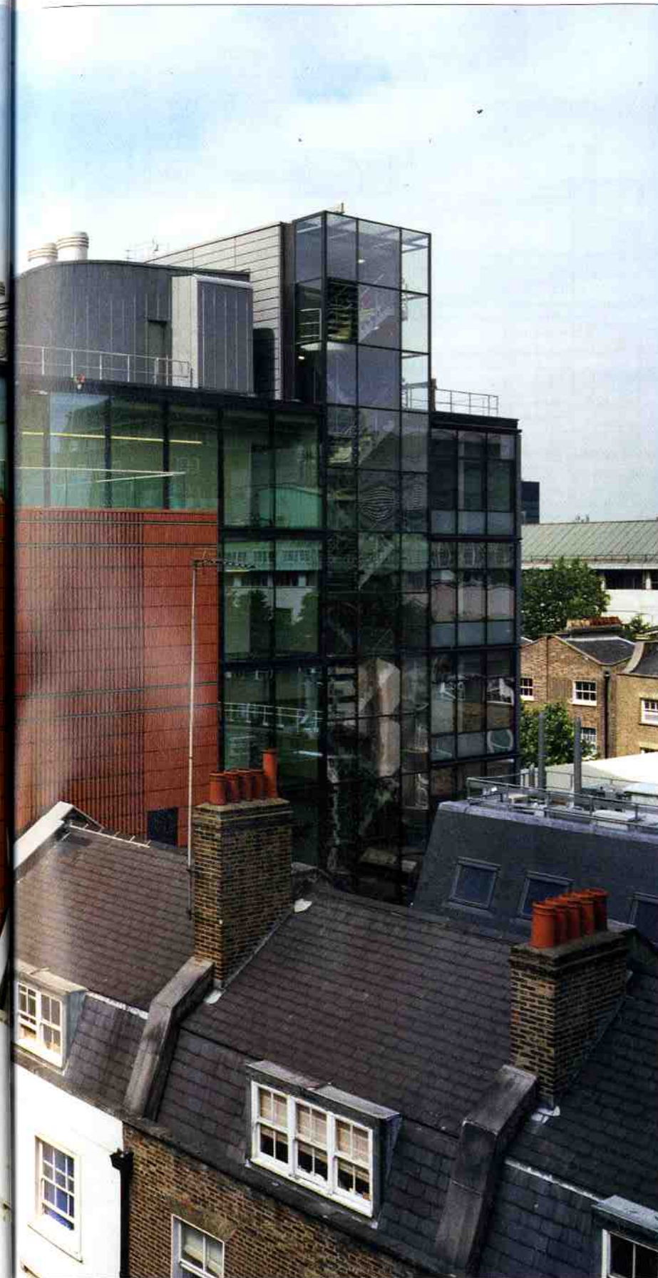
6. Terracotta louvres link the new building visually to the Paul Waterhouse block and the original hospital beyond
