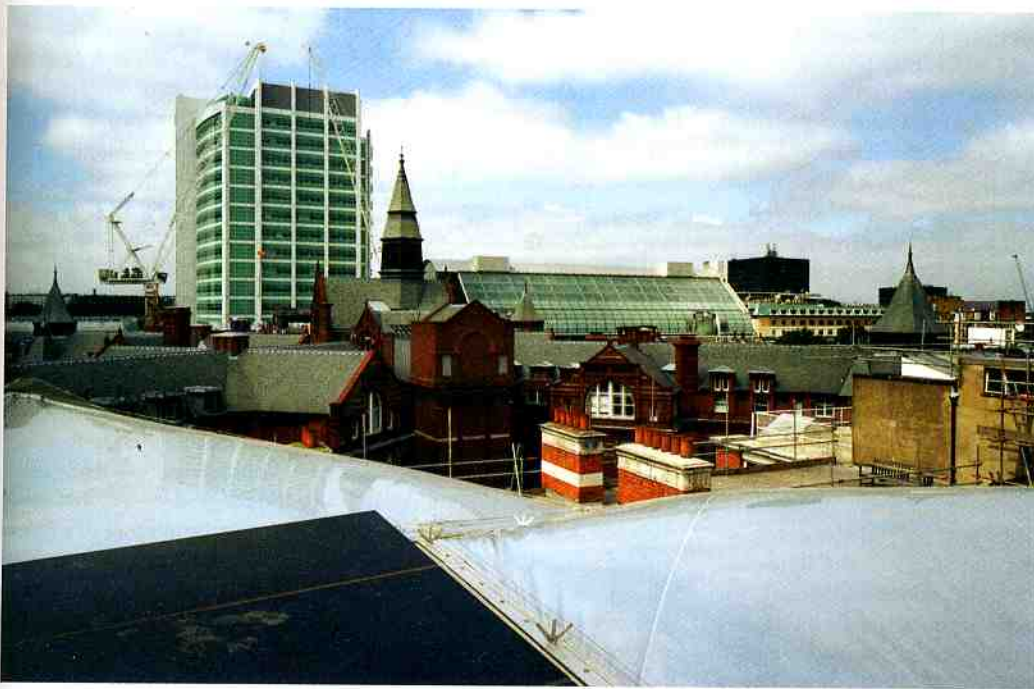
1. Rooftop view from the institute towards UCH's Euston Road Tower
