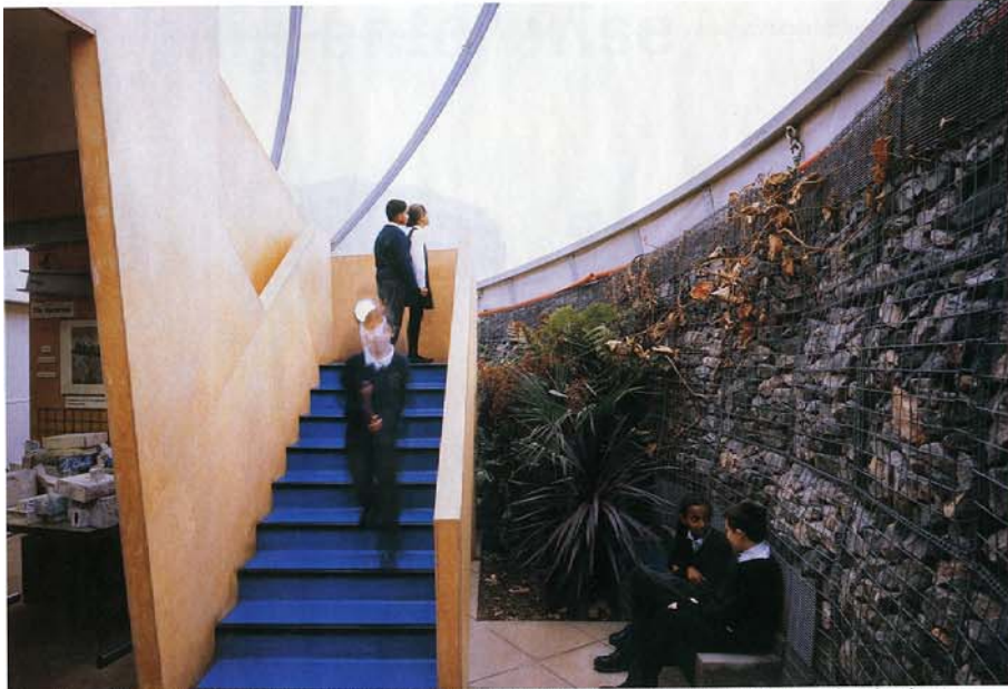
The gabion wall turns the building in on itself, leaving only hazy views out through the ETFE or distant images of the stars from the telescope.
