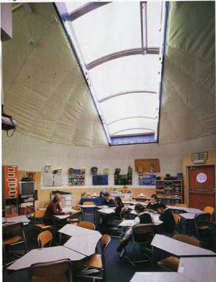
A rooflight cuts through the sailcloth ceiling of the pod.
