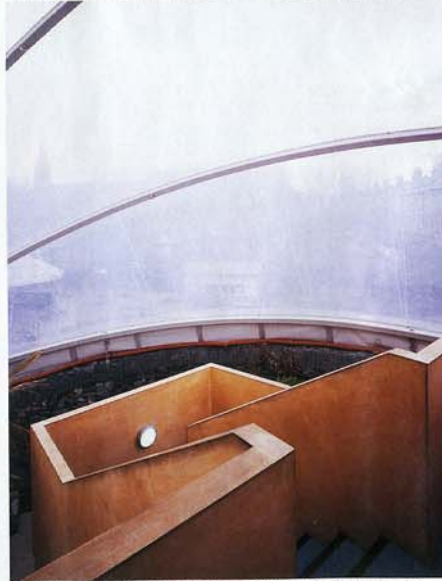
Plywood angles of the staircase sit against the curved conservatory.
