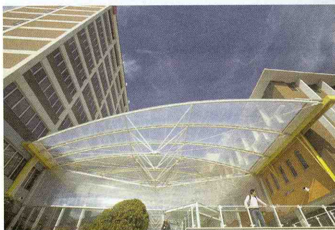
The ETFE atrium at Swinburne University, Melbourne, Australia.
