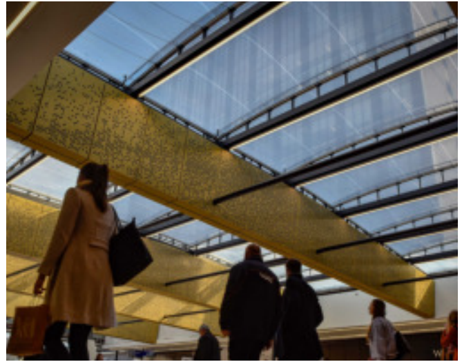
Installed PVDF Mesh to reduce rain noise, Leeds Train Station, © LeedsLive
